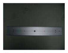
Using mounting bracket mark out fixing holes x6.
